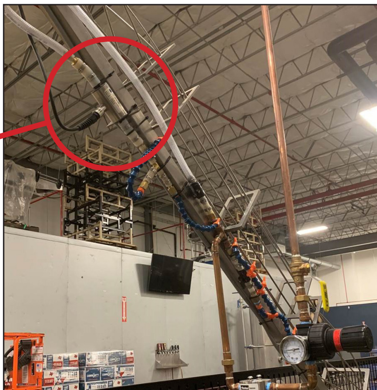
TAKK Inline Ionizer inserted into airline.
